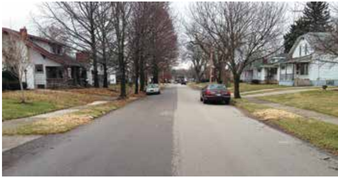
Maltene Rejuvenator: Sustainable Water-Resistant Performance. Image of Ohio roadway years after a maltene rejuvenator was applied and shortly after a rainfall. The treated section is dry, while the untreated section of pavement remains wet
